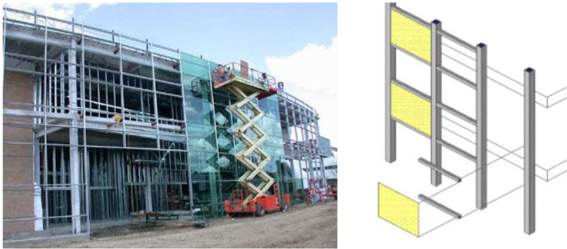
Figure 3. Stick Built Curtain Wall [9].
