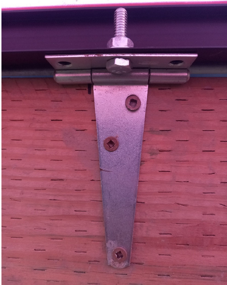
Figure 17. Hinge for changing the tilt angle of the module.
