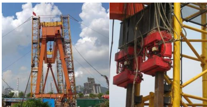
Figure 1. Hydraulic climbing system.
