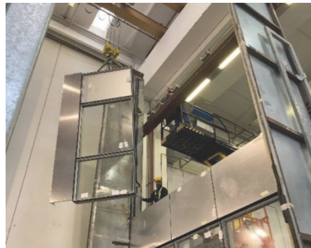
Figure 8. Façade installation process.
