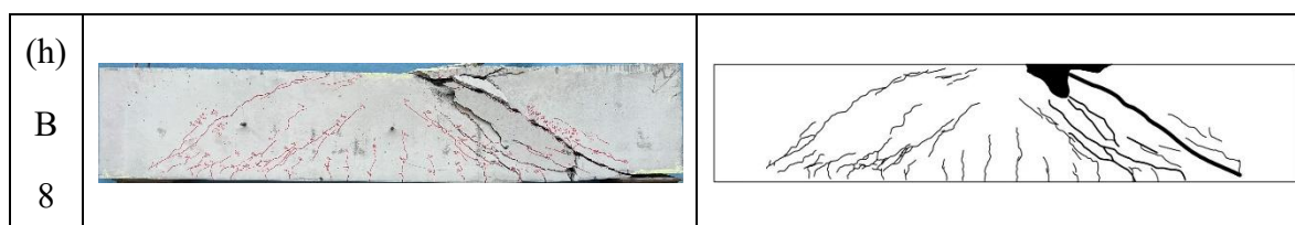
Figure 6. Crack pattern of each tested beam. (a) B1; (b) B2; (c) B3; (d) B4; (e) B5; (f) B6; (g) B7; (h) B8.
