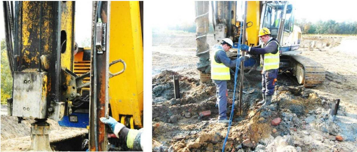
Figure 13. View of steel profiles with sensors during the insertion into the concrete mix.
