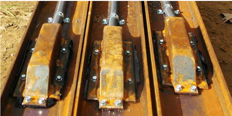
Figure 11. Protective casings installed on IPE120 profiles.
