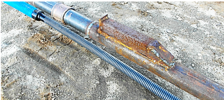
Figure 12. Protective casings installed on RO pipes 2"×2.9.
