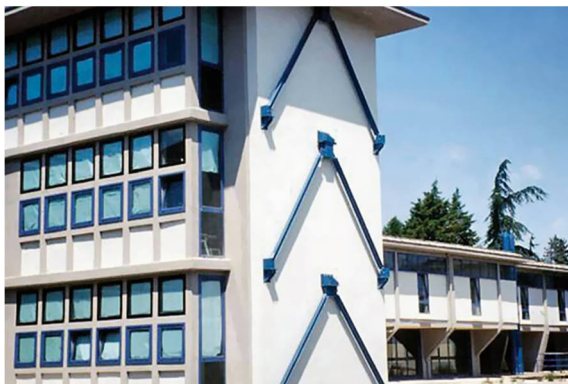
Figure 7. Retrofit intervention by means of viscoelastic dampers in the school Gentile-Fermi in Fabriano (Ancona) [58].
