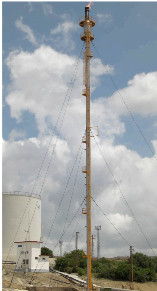
Photo 1: General view of a typical flare stack supported using guy wires
