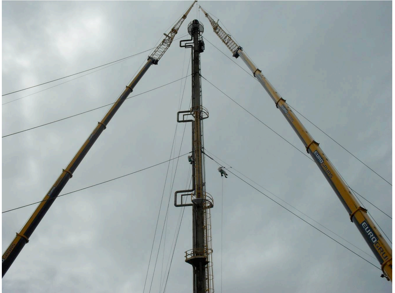
Fig. 02 Works on a flare stack using cranes and baskets, combined with rope access techniques for the inspection and lubrication of guy wires
