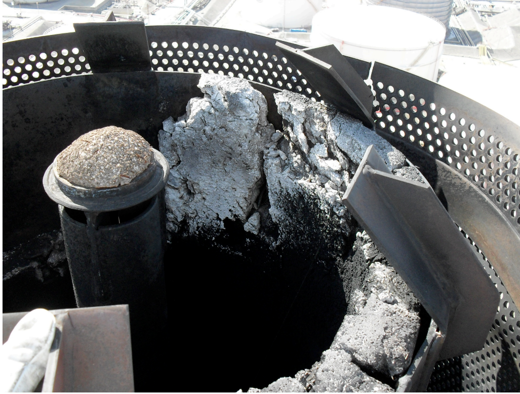
PHOTO 8.1 View from above of an installed burner, with detachment of fireproof coating
