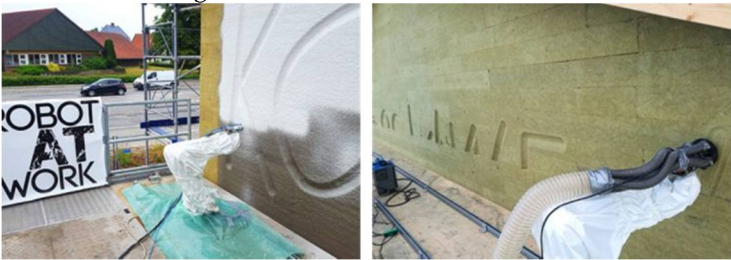
Figure 5. On-site 3D printing for renovation in Korslokke, Denmark [ http://www.robotatwork.com ].
