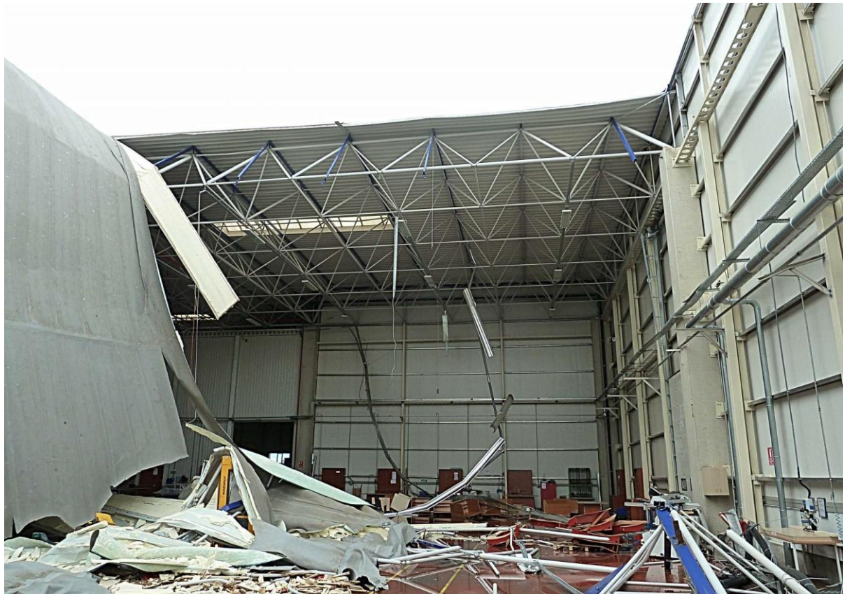
Figure 4. Damage on the roof of the space truss system.
