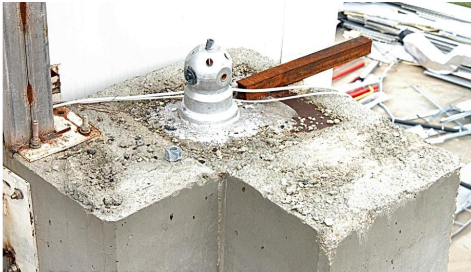
Figure 15. Damage on the support to which the space truss roof system is attached.
