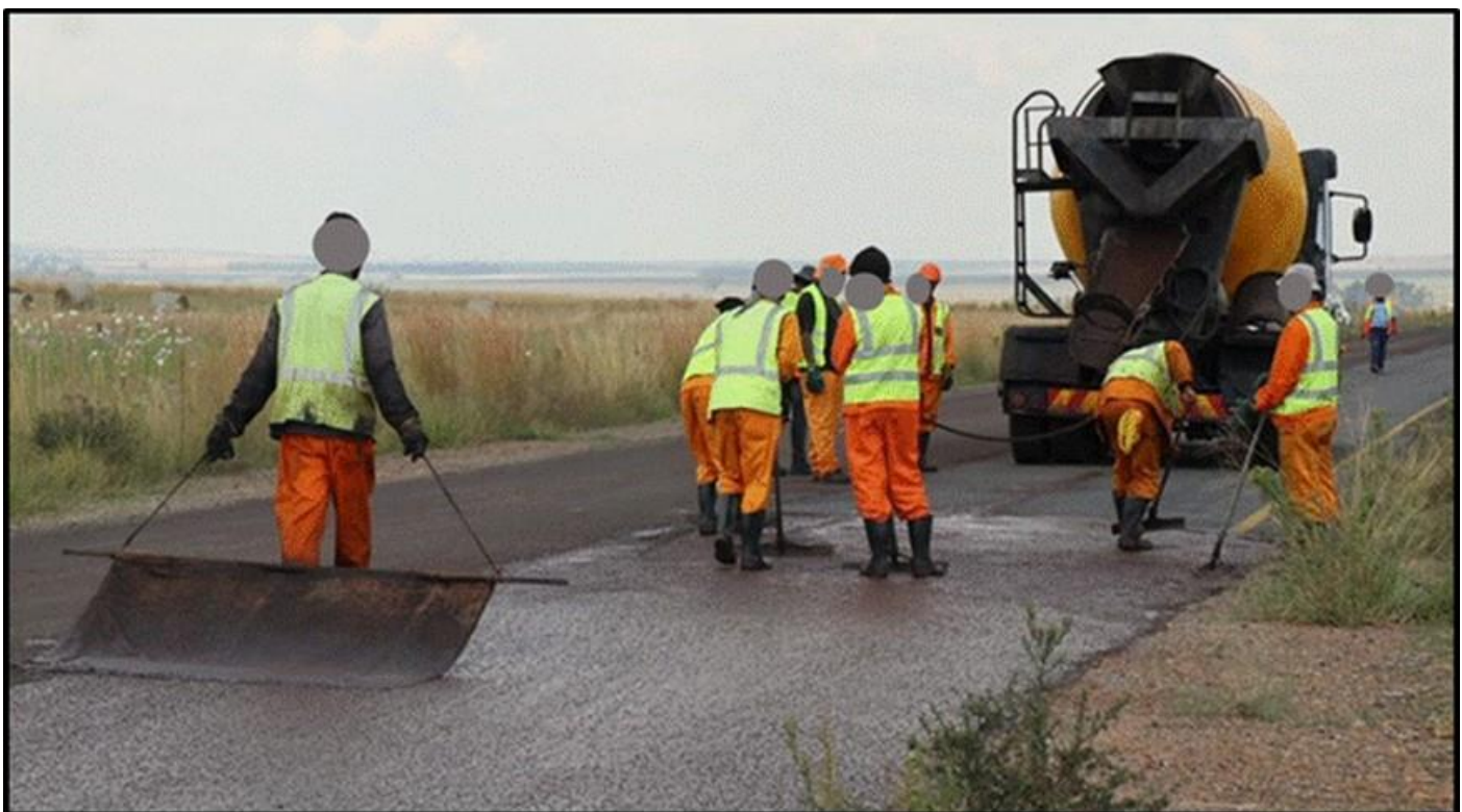
Figure 14: Slurry NME mix supplied to site using a large concrete mixer- spread and finished by hand.
