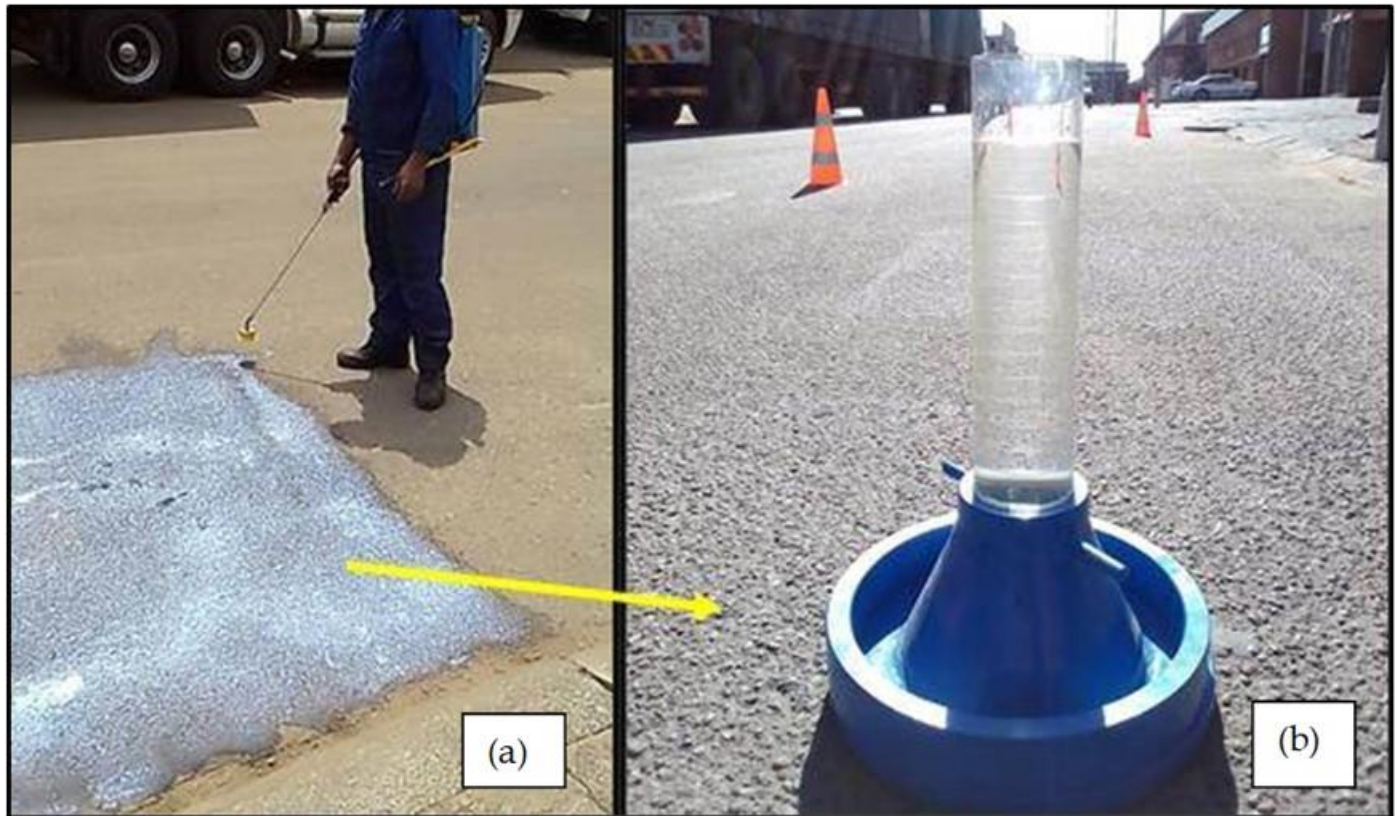
Figure 4: (a) Application of the clear-seal (5% NSNP diluted into water) (consisting of 50 per cent nano-polymer, 10 per cent nano-silane and 40 per cent water [18] ) by hand-sprayer at a rate of approximately 1 to 2 l/m 2 (about 5 to 10 ml of NSNP /m 2 at a material cost of about US$ 0.10 to US 0.20 /m 2 ); (b) the dried surfacing 30 minutes after application of the clear-seal with a Marvil apparatus placed on top of the surfacing to measure the rate of water penetration into the treated surface.
