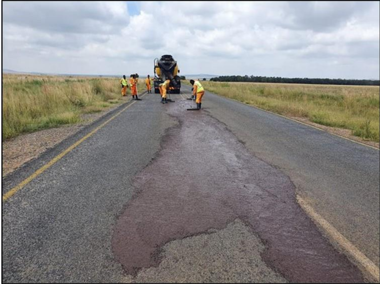
Figure 17: Filling of deformed areas on the road surface using a medium NME slurry mix as a pre-treatment to address severe deformation before applying a NME slurry across the whole lane as shown in Figures 13 and 14.
