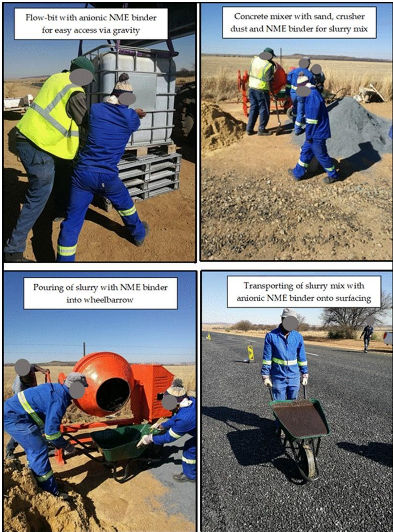
Figure 15: Labour-intensive road-side manufacturing of the slurry mix for a anionic NME binder slurry seal or for a modified Cape seal using an anionic NME binder
