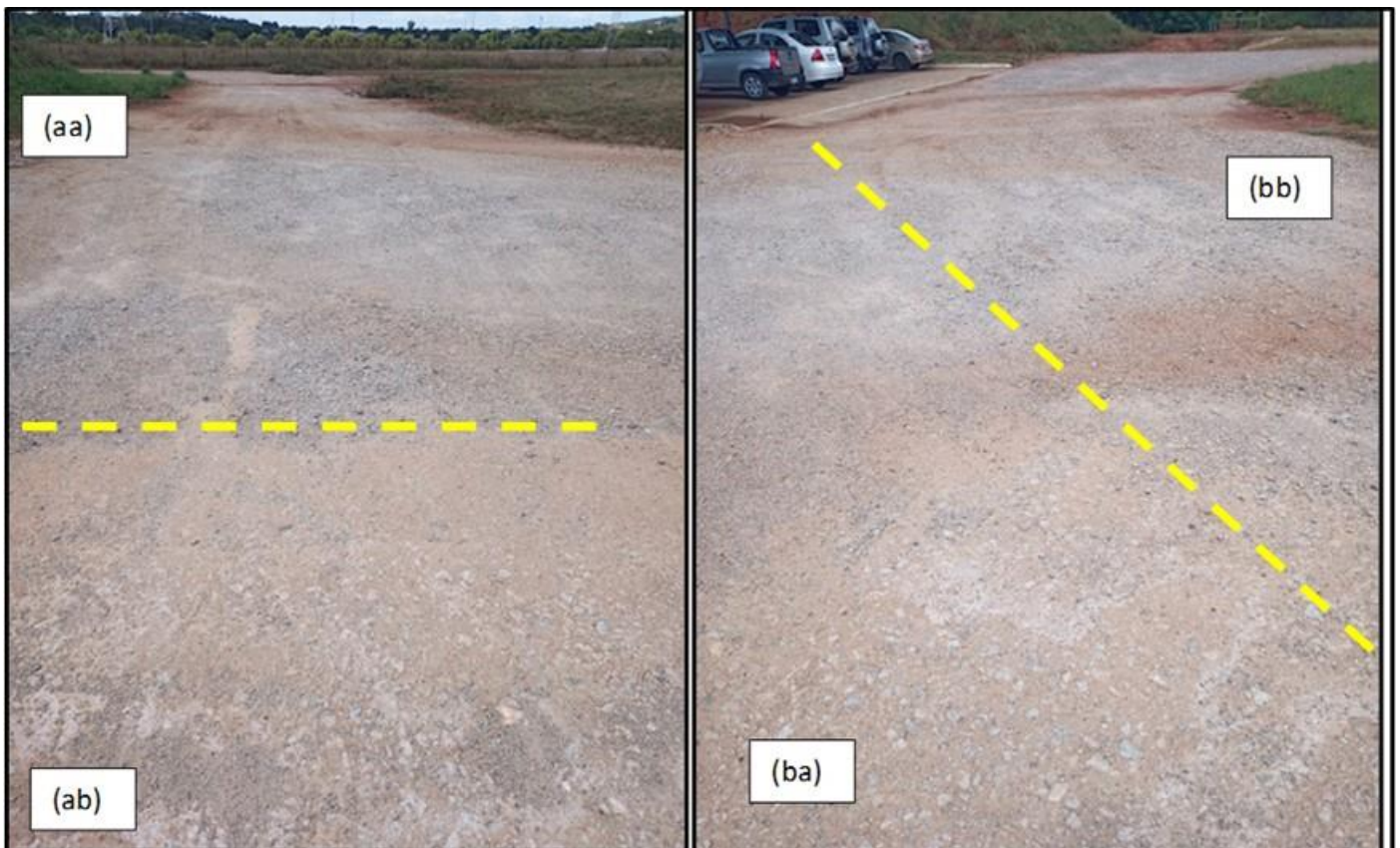
Figure 7: Condition of the G1[19] base-layer at the University of Pretoria, Engineering 4 facility after being open for 9 months from 21/8/2020 to 20/5/2021: (aa) Un-treated G1 layer subjected to rain; (ab) Clear-seal [18] treated subjected to rain; (ba) Clear-seal [18] treated subjected to rain; (bb) Clear-seal treated subjected to rain and light traffic
