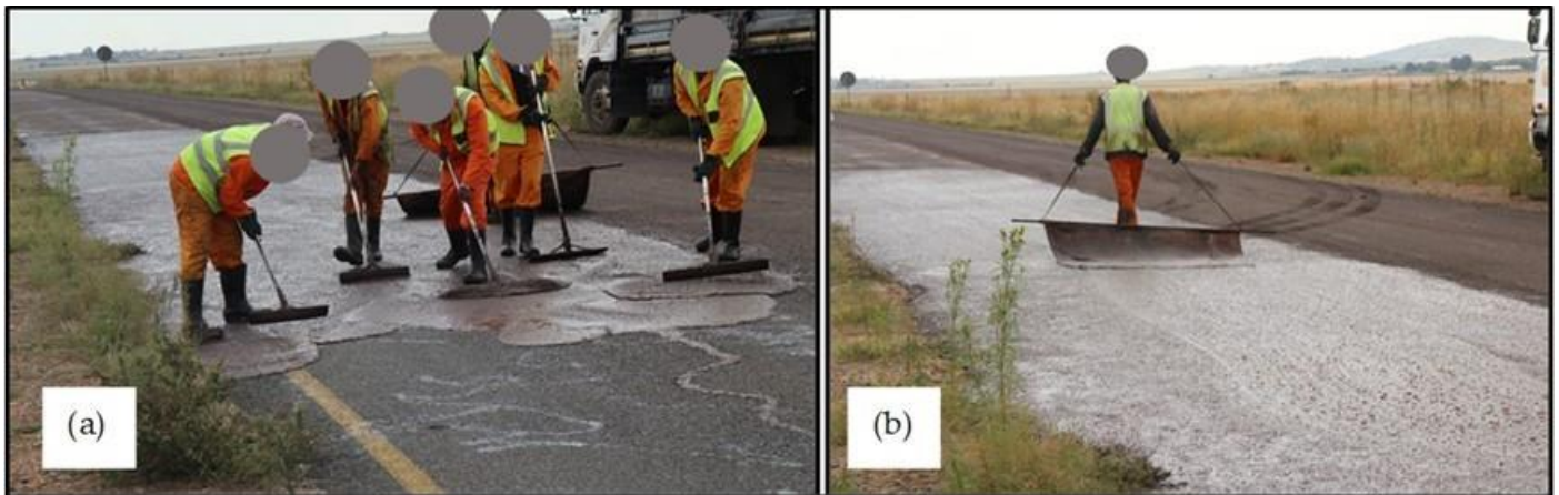
Figure 13: Application of a labour-intensive anionic NME slurry seal to effectively provide a water-repellent new surfacing, preventing water-ingress into the pavement structure on as severely cracked surfacing without disturbing the existing surfacing and restoring some riding quality – this surfacing will dry within 6 hours due to the water-repellent addition of the nano-silane – a six hour working envelope is created by dilution the anionic NME modified normal slurry mix by 50:50 with water, reducing the bitumen content by about 50% while creating a permanent bonding to the old surfacing and a water-resistant surfacing.
