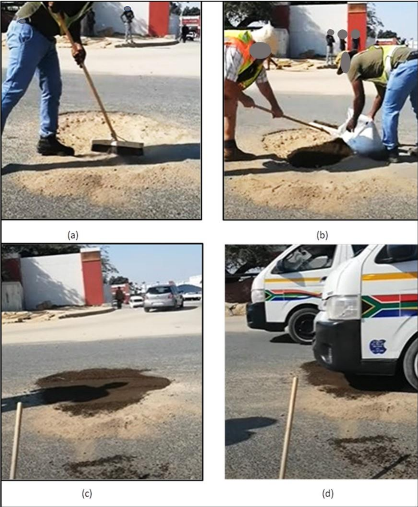
Figure 11: (a) Cleaning of pot-hole; (b) filling pot-hole with a water-resistant anionic NME gravel [24]; (c) hot-hole filled and partially compacted by hand, and (d) vehicles driving over filled pot-hole and increase compaction (Photographs provided and published with permission [20])
