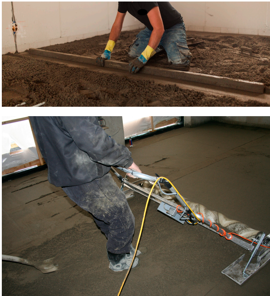
Figure 1. A sand-cement bound screed floor layer working (a) using the traditional working technique and (b) using the manually moved screed levelling machine.
