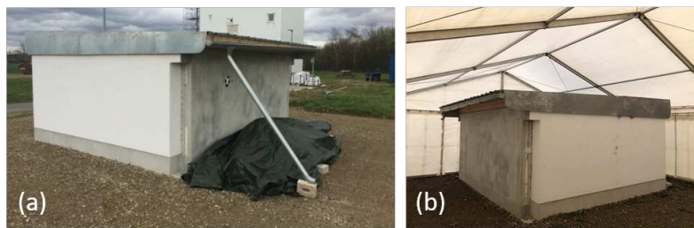
Figure 3. The test building without (a) and with covering tent (b).
