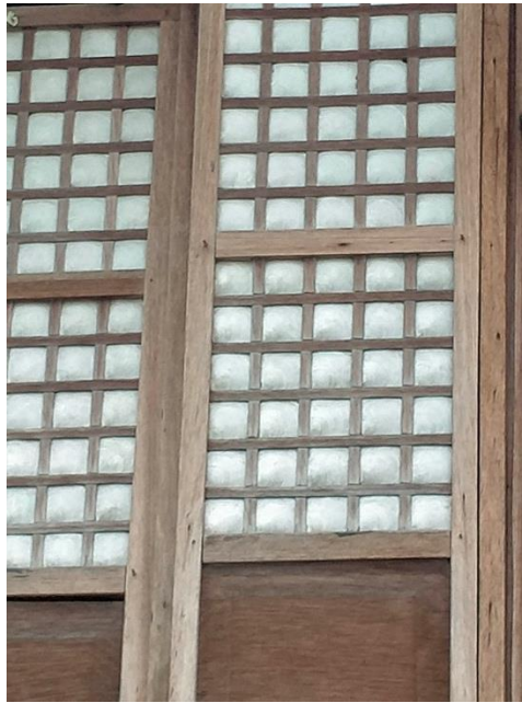
Figure 1. Example of a traditional Capiz window (photograph JMR, June 20,2023, Samal, Bataan, Region III, Philippines).
