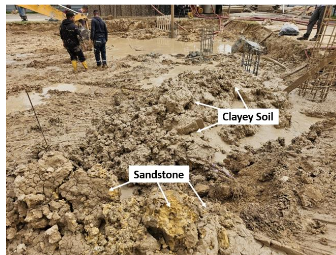
Figure 8. The photograph of the construction site under study during the pile drilling campaign. Wet brown clayey soil, stabilized with Bentonite, is visible on the surface. Extracted yellow sandstone at 9 meters corresponds accurately to GPR findings (Figures 6 and 7), affirming the reliability of aerial GPR for subsurface mapping in foundation engineering.
