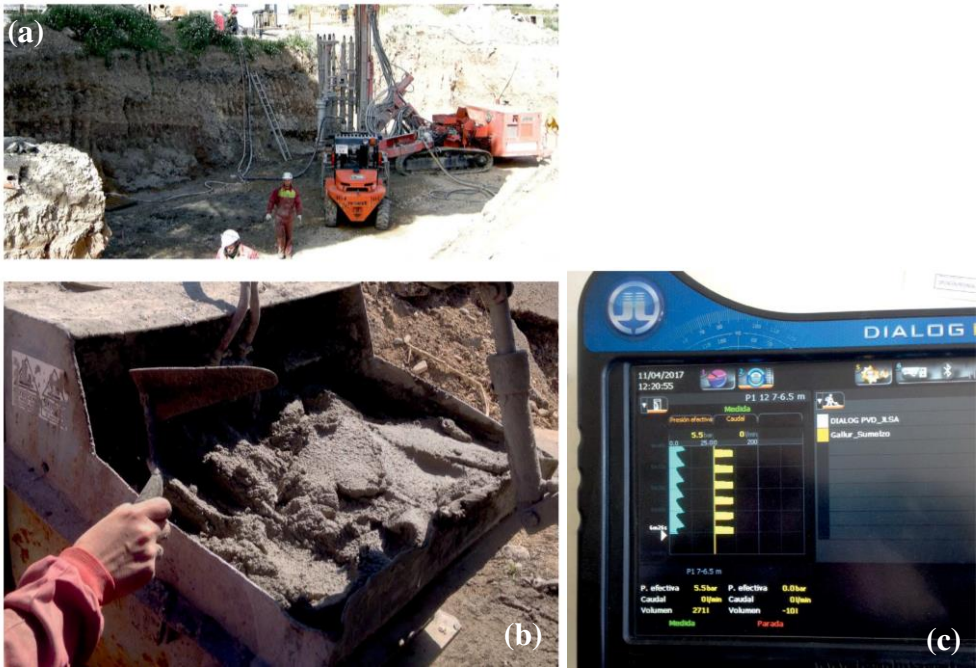
Figure 10. (a) Drilling equipment located in the excavation made at -3.00 m from the original street surface; (b) Appearance (texture and consistency) of the injection mortar in the injection pump hopper; (c) Injection control equipment: Injection in the interval between -7.00 and -6.50m; Effective pressure at that time 5.5 bar; mortar intake volume, after 6.26 minutes: 271 l.
