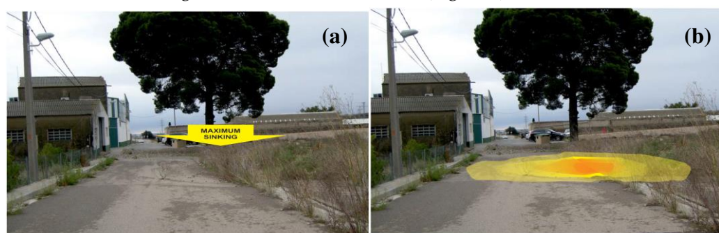
Figure 1. Panoramic image of the apparent subsidence of the road surface of the access to Gallur along the Camino Real (2015). The most depressed area is highlighted in color. This access had remained closed for several years.
