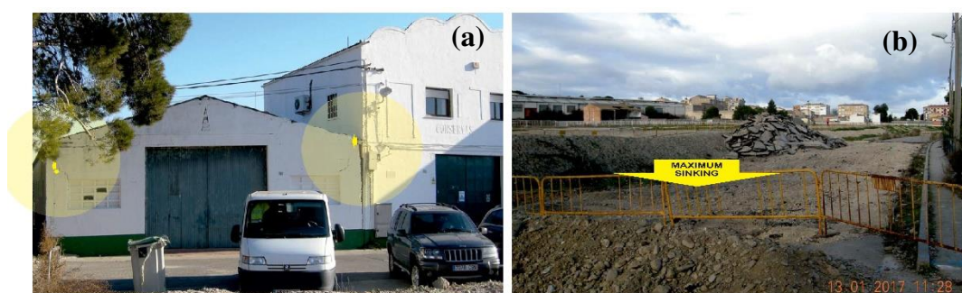
Figure 7. (a) Damage to an adjacent building is evident, highlighting points where deformations (cracks) are most pronounced, along with their indicated direction. (b) View of the street affected by the subsidence where the maximum subsidence is marked.
