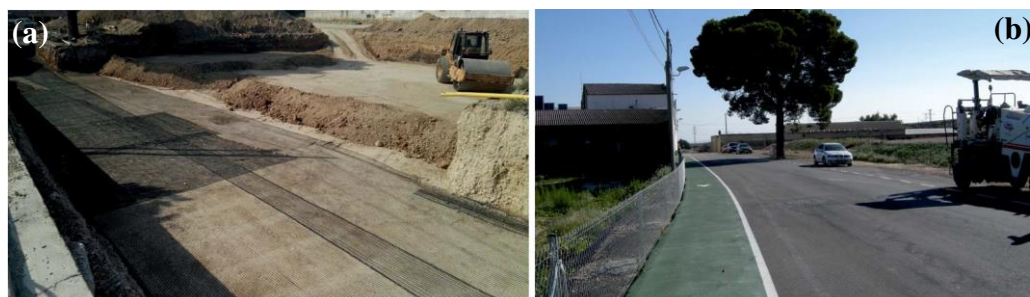
Figure 14. (a) Construction of the backfill with granular material; (b) Final state of the area after treatment and asphaltting.
