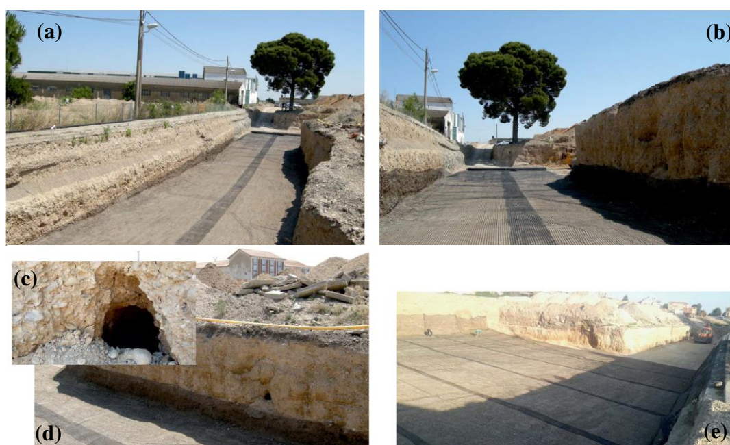
Figure 13. Photographs showing part of the reinforced backfill solution shown in Figure 12: (a) and (b) Longitudinal profile area; (c), (d) and (e) Transverse profile area. Figure (c) shows in detail a karstic cavity detected during the treatment.
