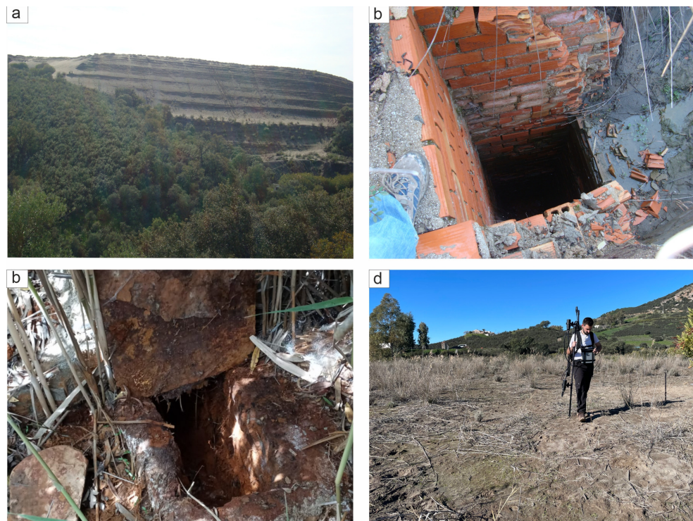
Figure 2. Photographs. (a) General view of the tailings dam. (b) Upper part of the chimney drain installed in the dam. (c) Details of the drainage at the foot of the dam. (d) Field procedure used for magnetic data collection.
