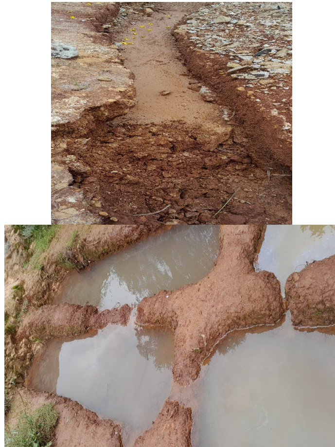
Figure 10. cut-off drain the wrong size and destroyed. Source; Horticulture and Conservation Department, Gullele Botanical Garden, 2023.
