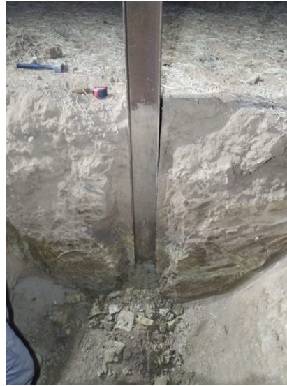
Figure 6. Unraveling the soil-pile bond. Permanent deflection and separation for FT-3.
