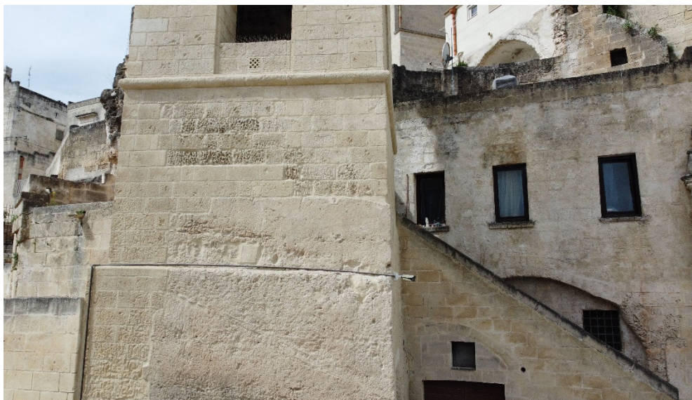
Figure 3. Detail of the bell tower of the rupestrian church of San Pietro Barisano. The deterioration of 'calcarenite' can be seen in several areas.
